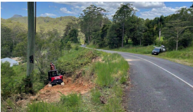
Image: Putting in an access track to investigate landslide damage
