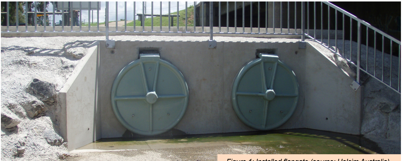
Figure 1: Installed flapgate (source: Holcim Australia)
